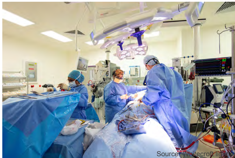
Example of a lighting installation in a healthcare environment
